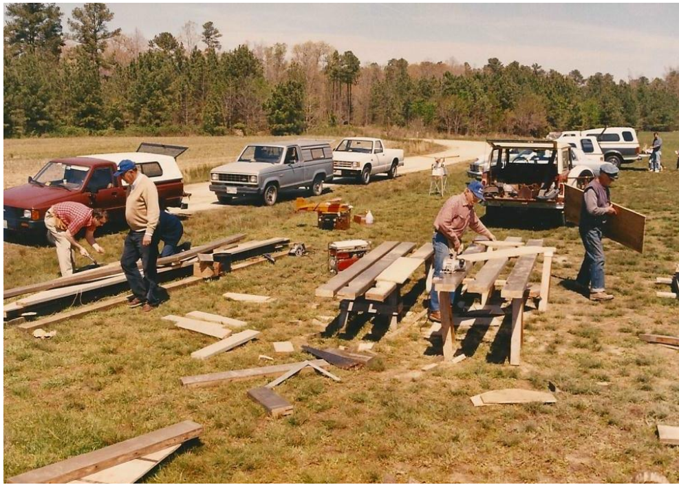
Shelter materials finally arrive and construction begins.
