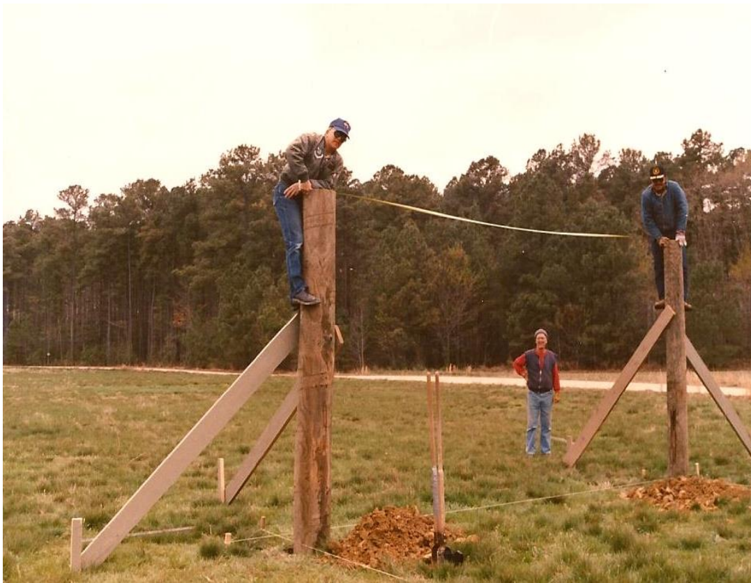
After a couple of months of work, we had our picnic shelter. Here, Carl Purgold and Julian Harris do the post leveling work.
